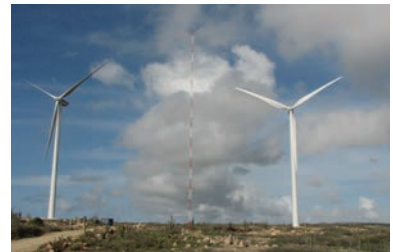
Wind resource assessment on Aruba
