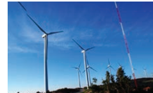
Wind Farm Monitoring (SCADA)
